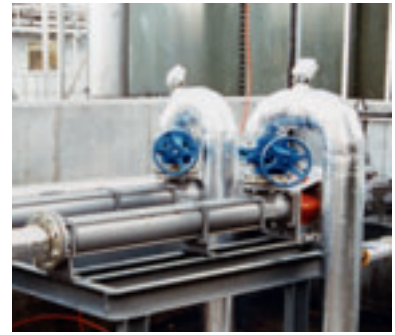
Pumping of slurry mix
